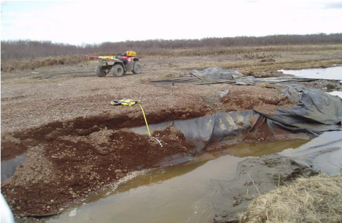
Photo 2: Airport Way Erosion / Washout, May 2005.
