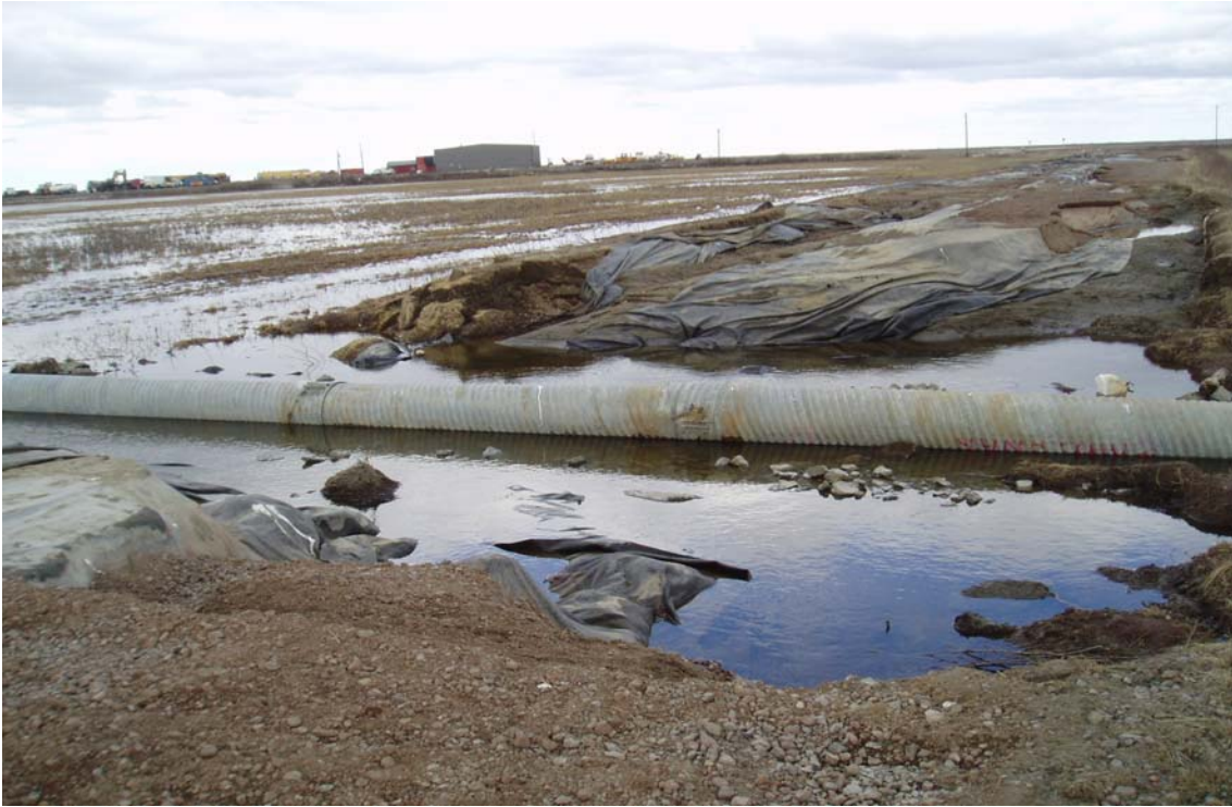
Photo 1: Airport Way Washout and Exposed Culvert, May 2005.
